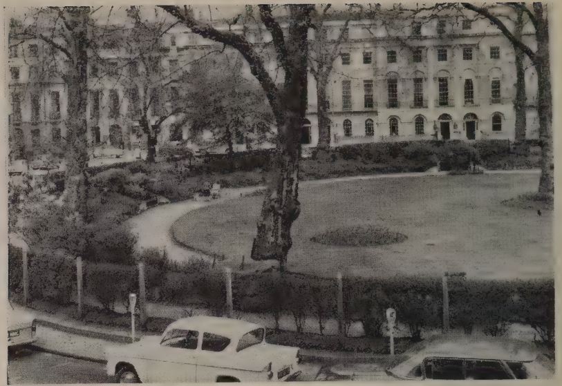
201 Fitzroy Square. The square and the surrounding buildings form a valuable group worthy of preservation.
